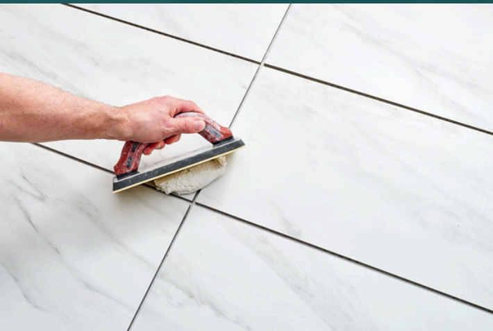
Sealer Grout Applying on Tile
